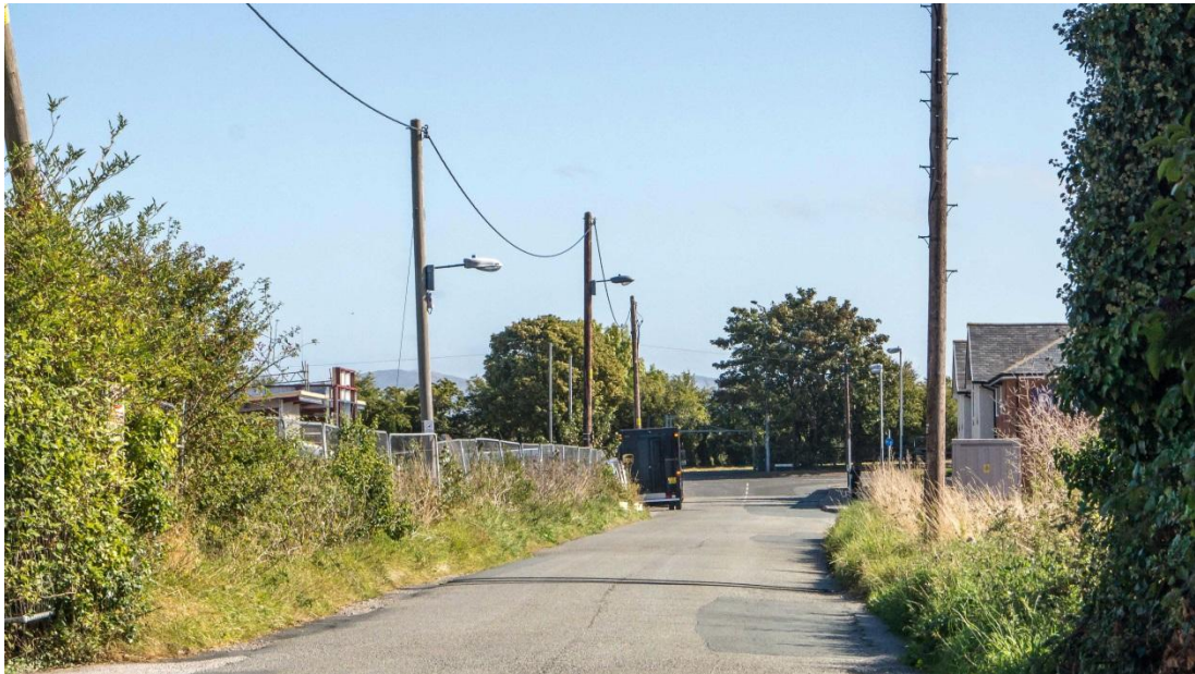
7.6 Photo 8 View along Marsh Road towards Station Road (September 2014)
